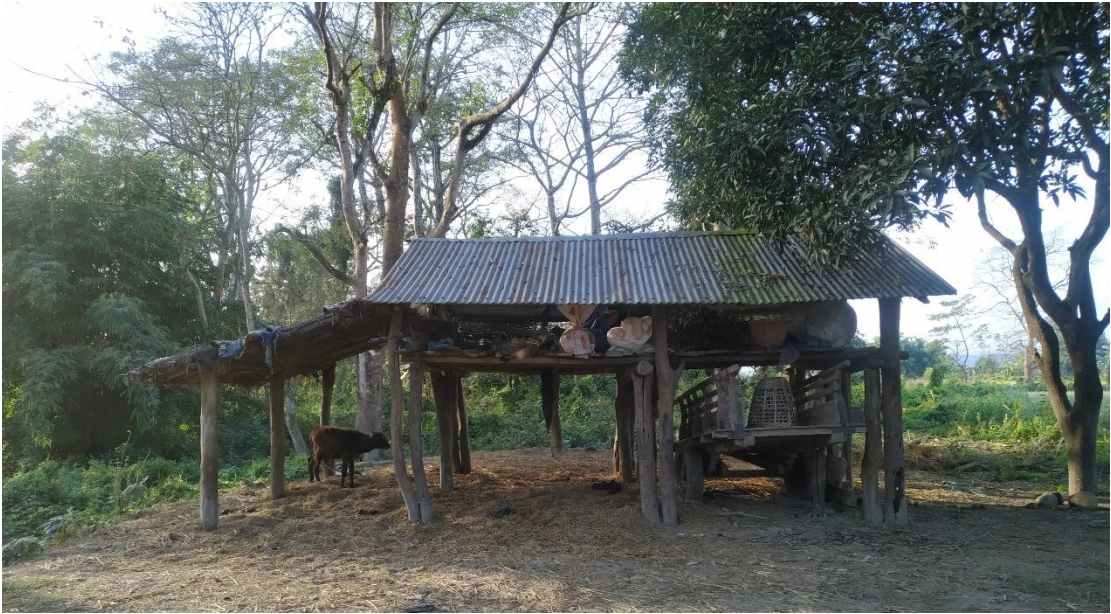
Figure 13: A cattle shed with the lower level for cattle and carts, and the upper level for storage - generally agricultural tools, hays and fodders.
