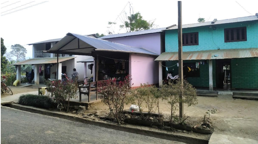
Figure 32: A cluster of ek dine ghar with front yards connecting the houses to the main village lane in the Charghare Tole. The house in the middle features a shop encroached in the front yard.
