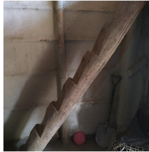
Figure 23: Steps are carved inside a timber log for ladder in the Mahato family's house.
