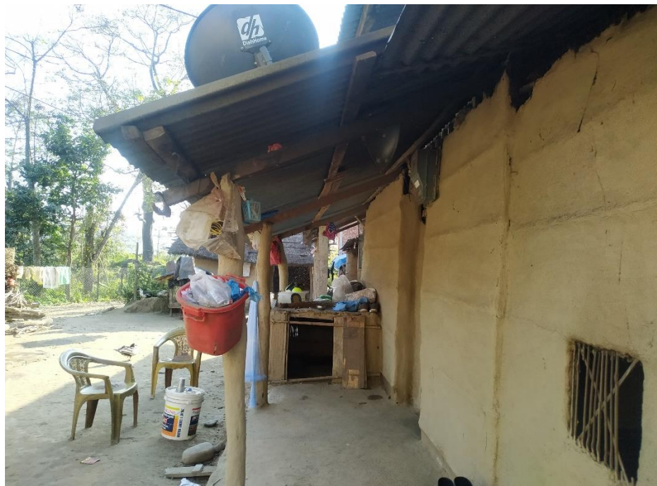
Figure 22: A porch buffers the interior with the outside in the Mahato family's in the Bhutaha Tole. An end of the porch is occupied by a poultry coop, dustbins, toothpastes, brushes, fishing nets and other daily tools are hung on the timber posts or the rafters. Plastic chairs from the market are offered to the guests for sitting in the front yard.
