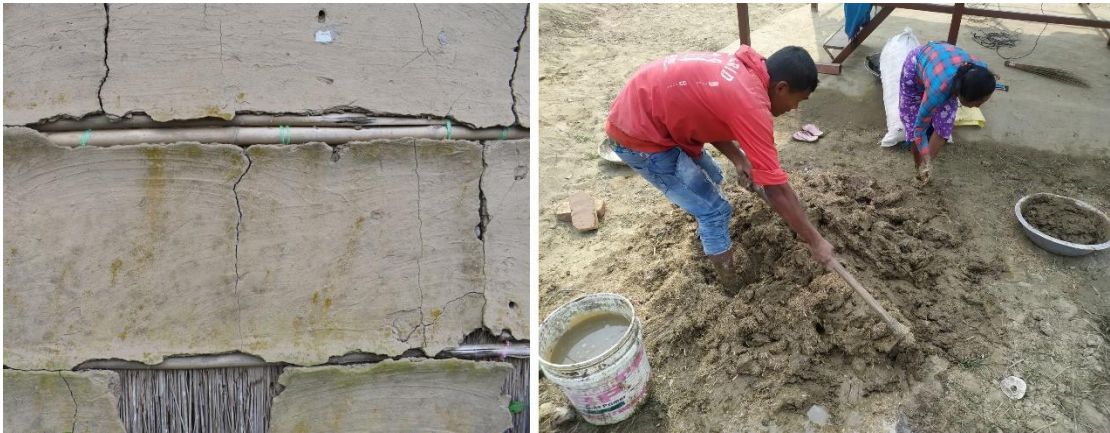
Figure 29: Right - mud mixture cladded on the tha: tha: ra to form walls get infested with molds and algae over time due to humid environment. Left - villagers stomp and mix mainly earth, dung, hay fibers to form mud slurry for the wattle-daub walls.
