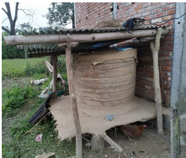
Figure 37: Granary made of flattened bamboo mat raised on stilts and covered with tin sheets found behind an ek dine ghar in the Charghare Tole.
