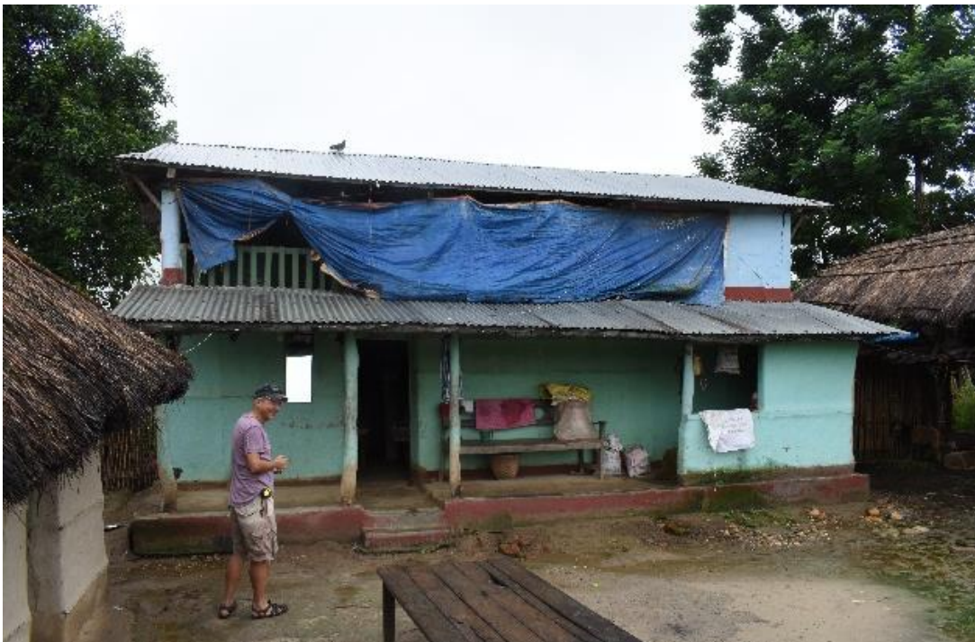
Figure 25: A double storey traditional Tharu house belonging to a Thanet family in the Hetki Tole . It hosts living arrangements for a joint family of ten. Kitchen and dining is in the hut to the left in front of the building. The balcony is covered with a tarpaulin to prevent from rain.
