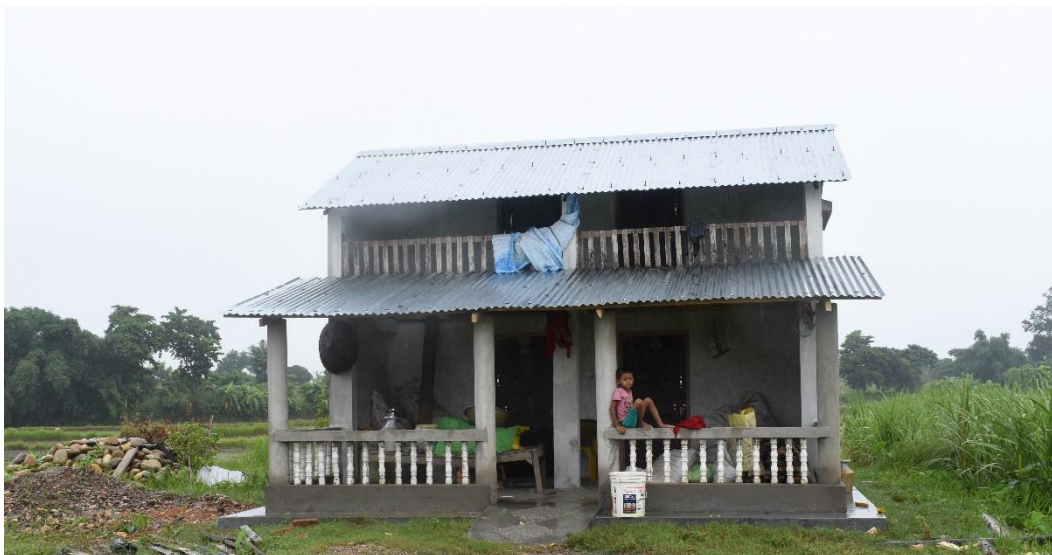
Figure 35: A newly constructed ek dine ghar at the Hetki Tole boasts a front porch which leads to two rooms at the rear end of the house. A wooden ladder leads to the upper floor.
