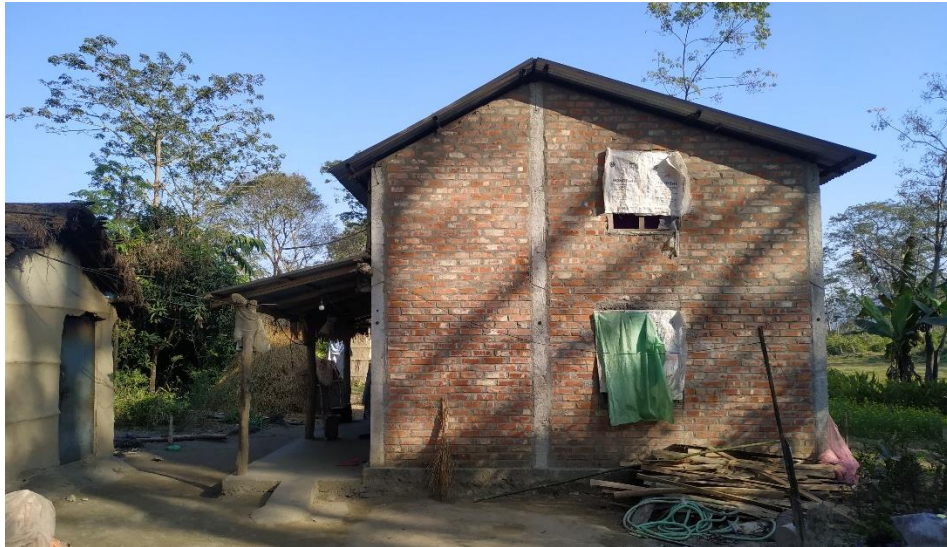
Figure 36: Ek dine ghar found in the Bhutaha Tole is accompanied by a hut built in old traditional style which houses kitchen dining. Synthetic granary bags are cut and used to cover the timber frames in the openings.
