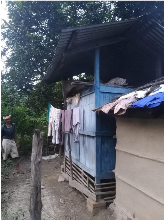
Figure 16: Typical structures of timber raised on stilts with tin sheets roofing can be found in the village which is used to store granaries.
