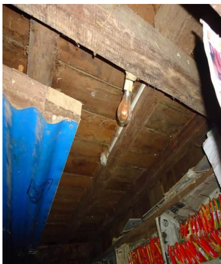
Bulb lighting due to power of MHP
