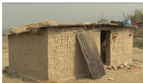
Figure 20. Labor's home in brick kilns
