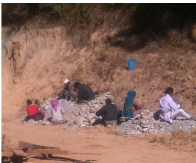
Picture 6.2 Construction Workers
